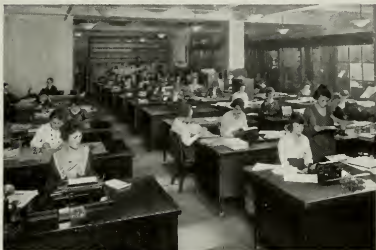
Main Office, Ninth Floor, Home Office
