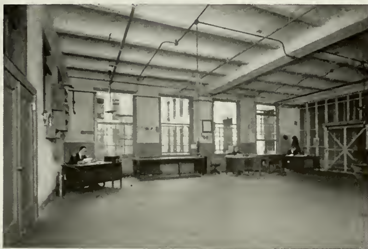
Interior of Warehouse
