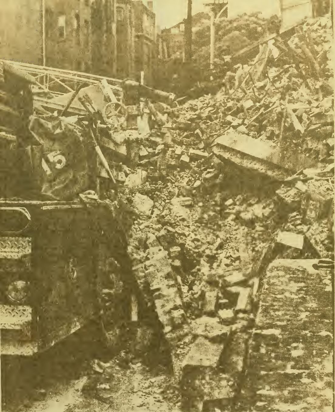
LOWER PORTIONS OF E-LINE WALL LYING AGAINST LADDER TRUCK 15
