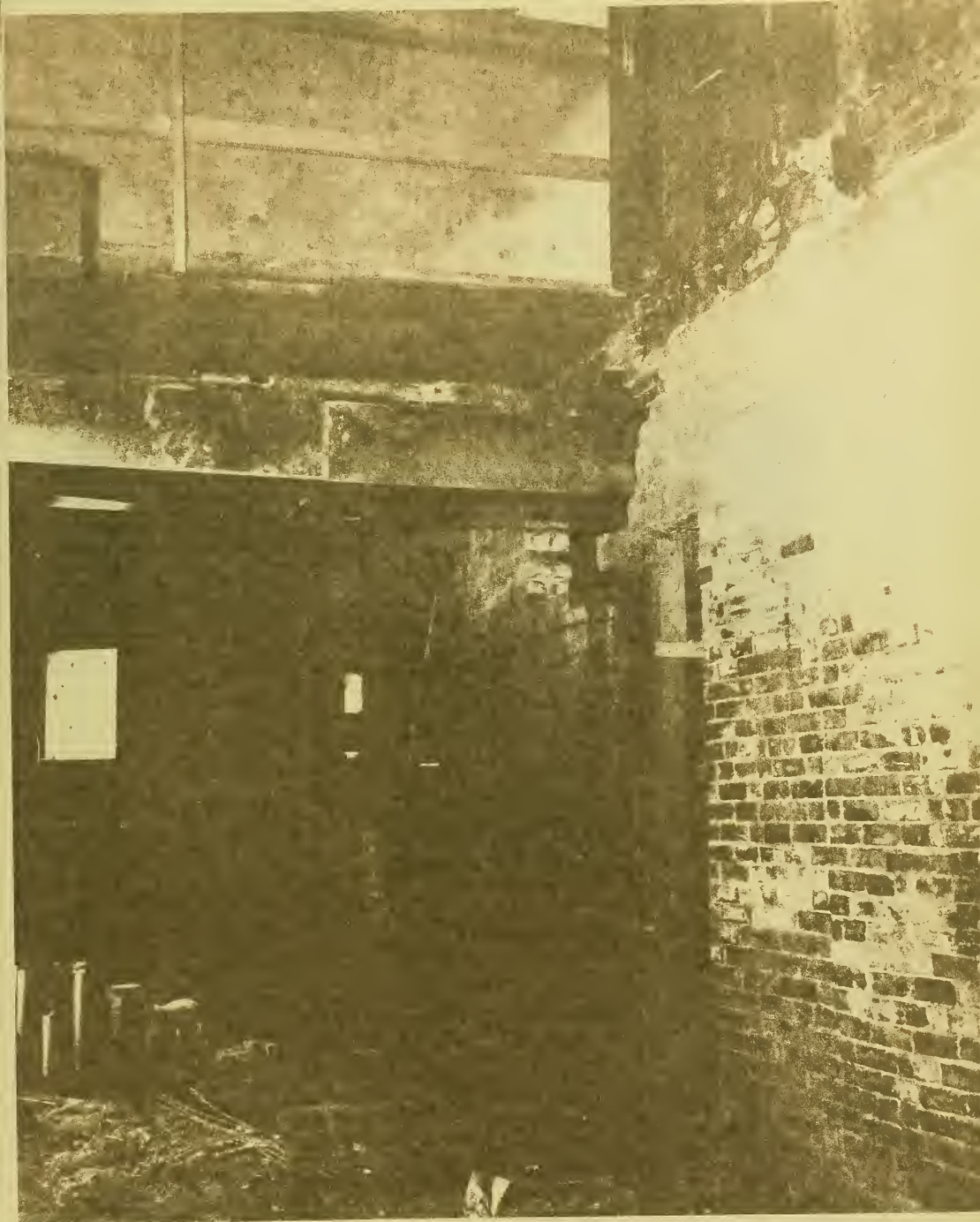
SHEET METAL DUCT PASSING THROUGH B-LINE WALL (PHOTO TAKEN SOMETIME BEFORE COLLAPSE)
